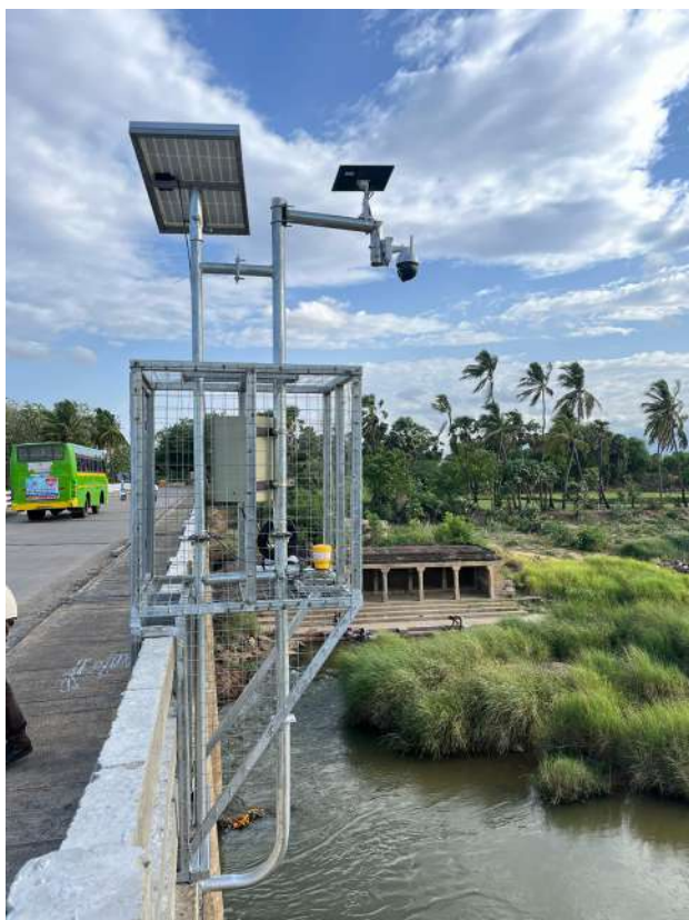
March 2025, Tirunelveli: Tirunelveli has implemented a flood early warning system, which is equipped with upstream and downstream sensors feeding into a centralised monitoring hub.
